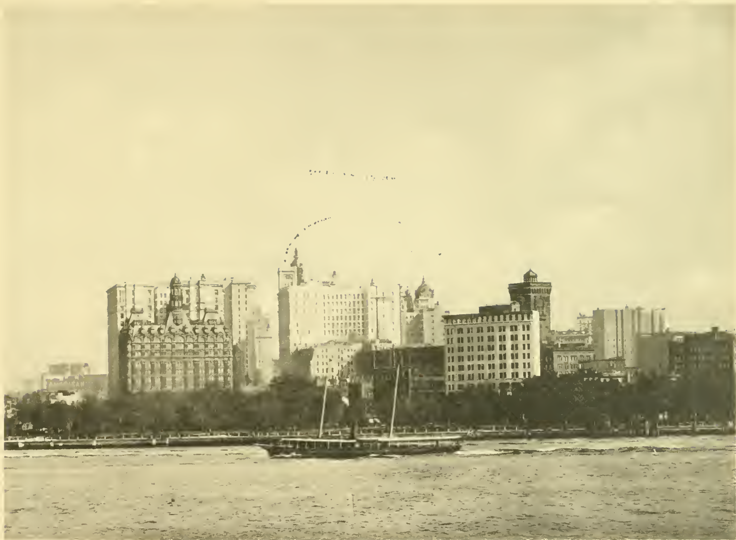
Bowling Green Building, Washington Building.
